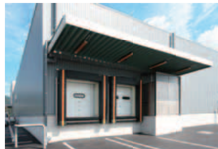
Dock shelter / Overhead door
